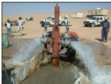
Specially designed wellheads were made to contain the high artesian pressures.
