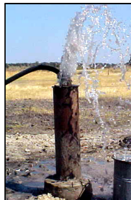
After drilling, monitoring boreholes were developed using compressed air jetting.
