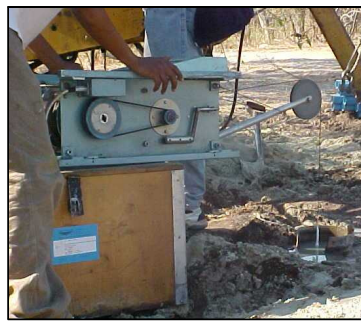
After completion of drilling, a downhole logging probe is lowered in to the borehole to measure the properties of underground formations, which provide useful information for borehole design (placement of screens).
