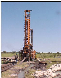
Exploration borehole drilling using Reverse Fluid Circulation (RC) Method.
